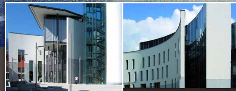
CITY HALL Brunico Architect: Abram / Schnabl Company: Gasser
